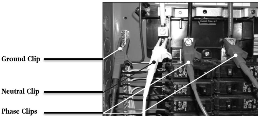
Single phase shown, third phase would require the third phase clip to be connected
