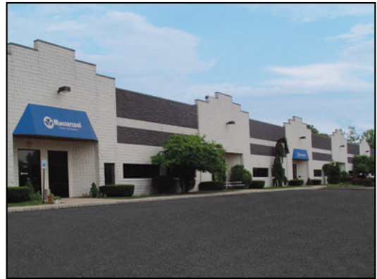
European Sales Office and Warehouse
