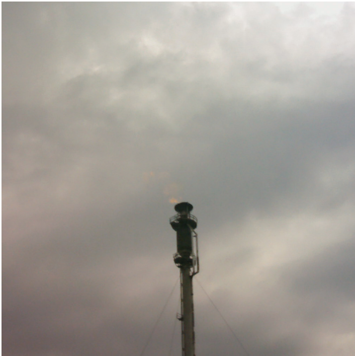
A flare stack with a small flame coming out on a cloudy day
