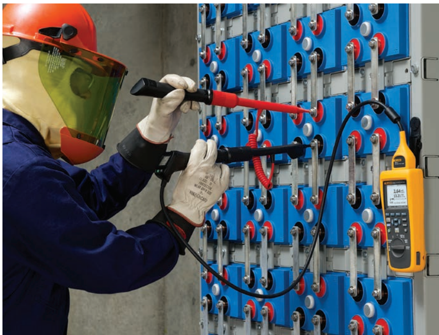
Measuring ohmic values in sequence mode
