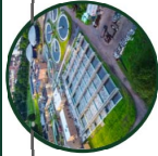
Water Treatment Plants
