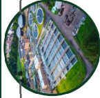
Water Treatment Plants
