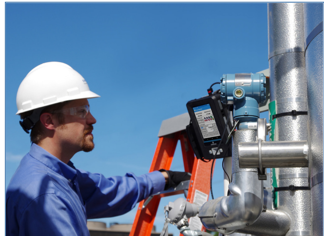
The magnetic hanger accessory allows you to attach the Trex unit to a pipe, freeing up your hands for other work.
